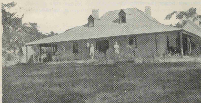
HUME'S HOUSE, YOUNG.
